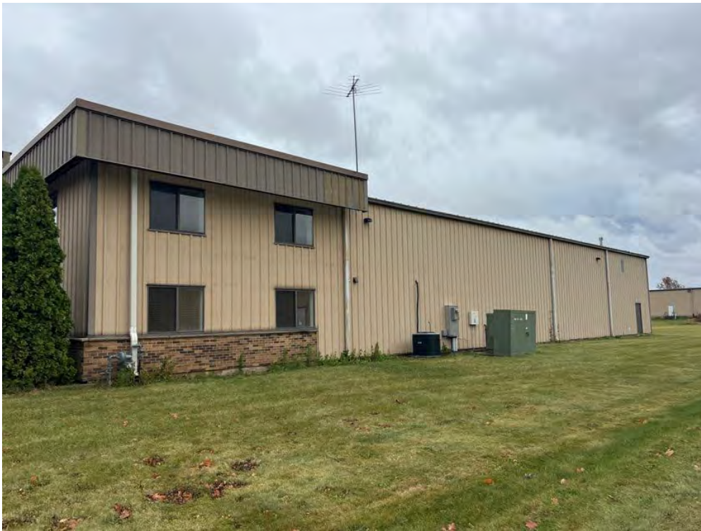
Photo 2 - View of the south side of the building, facing northeast.
