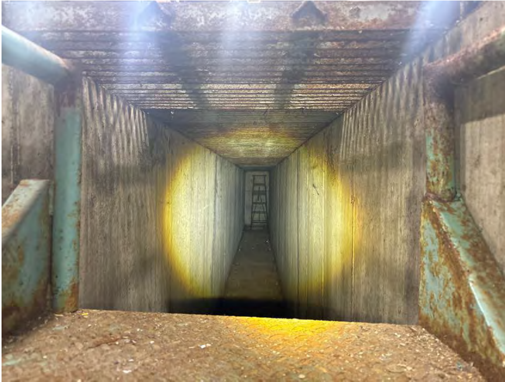
Photo 13 - View of the vehicle inspection pit in the warehouse.
