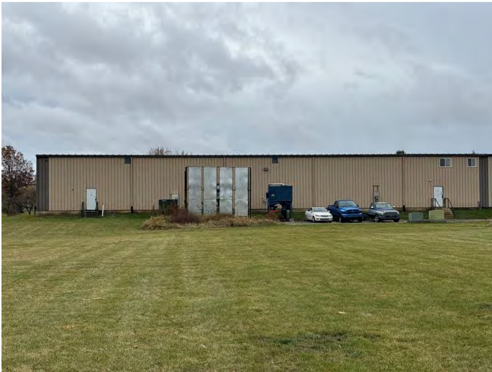
Photo 26 - View of the east adjoining property.
