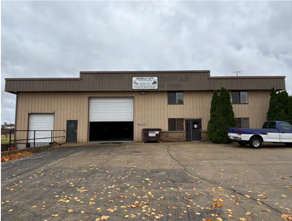
Photo 3 - View of the west side of the building, facing east.
