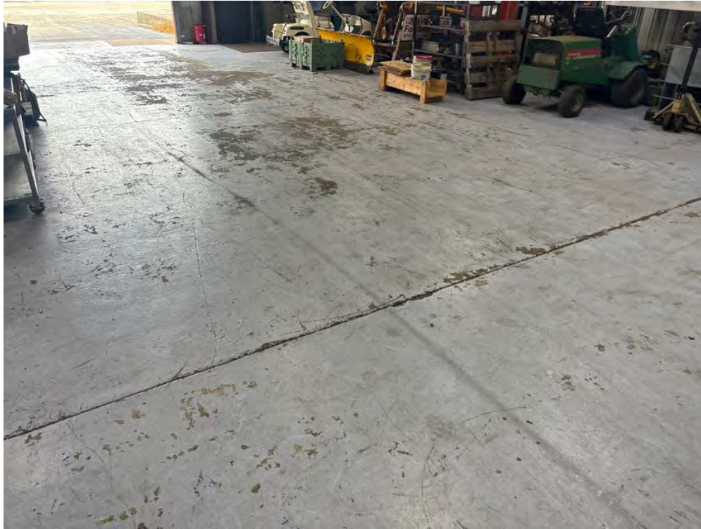
Photo 11 - View of the warehouse floor.
