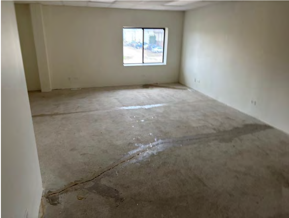
Photo 7 - View of the second floor office space.
