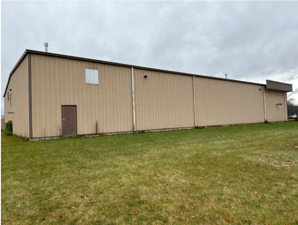
Photo 1 - View of the north side of the building, facing southwest.
