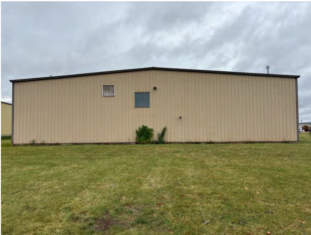
Photo 4 - View of the east side of the building, facing west.
