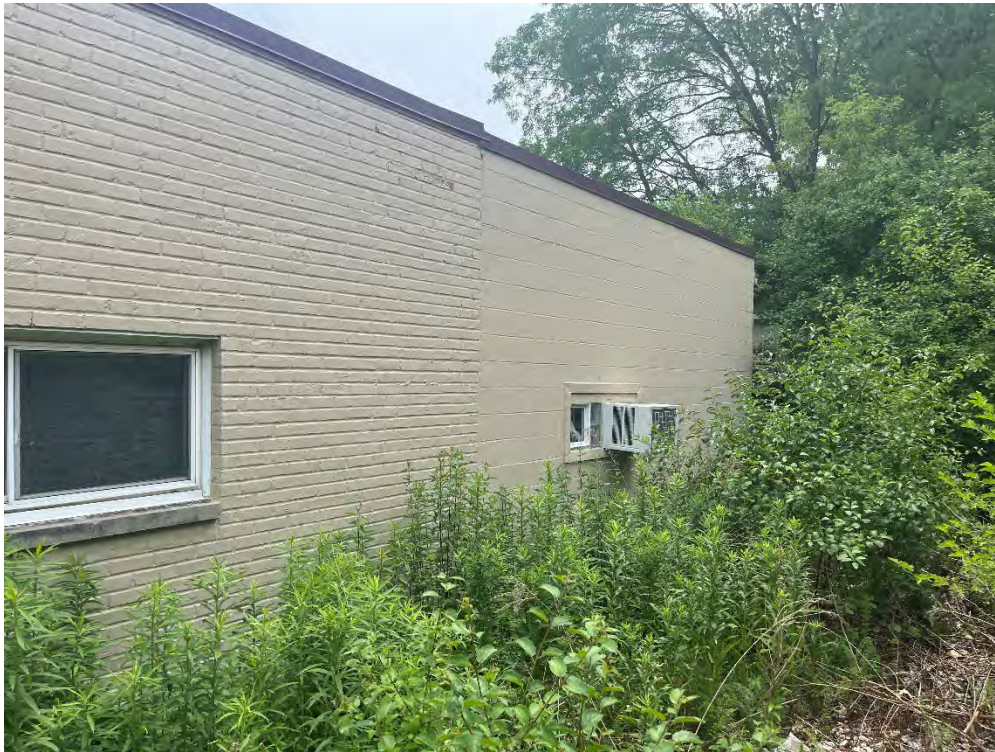
Photo 4 - View of the west side of the Subject Property, facing south.
