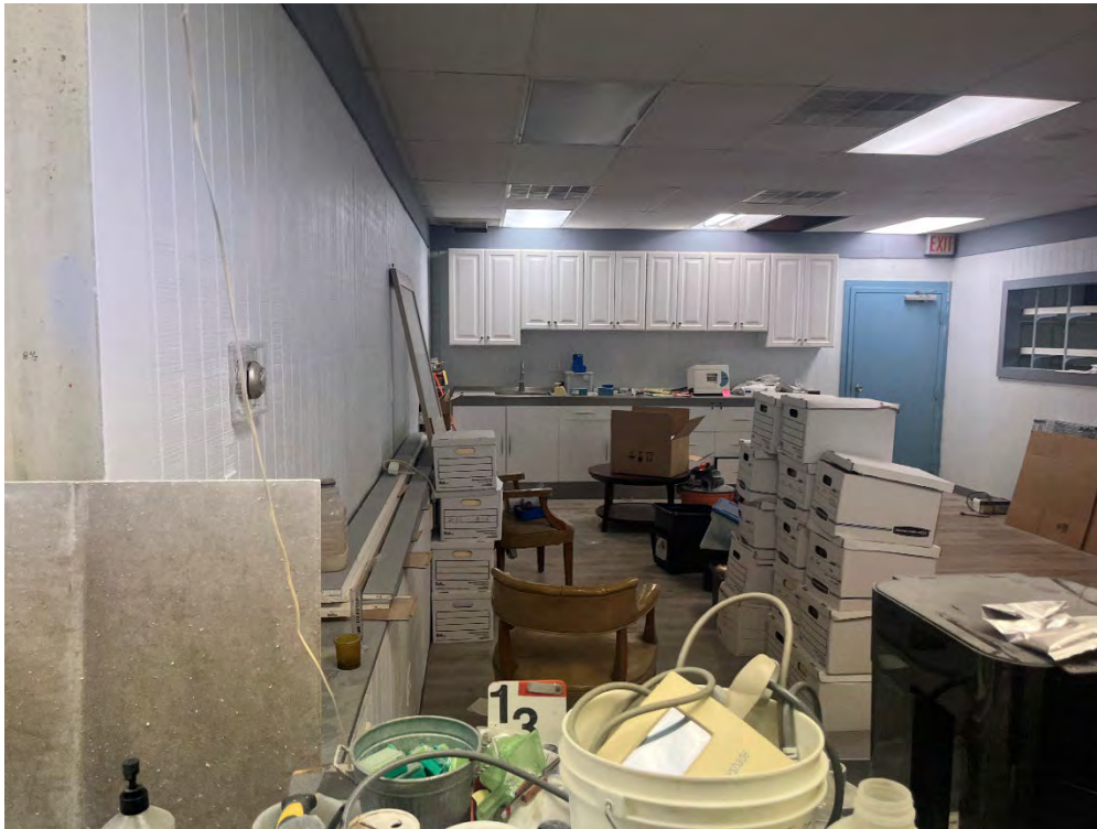
Photo 10 - View of a former office area.
