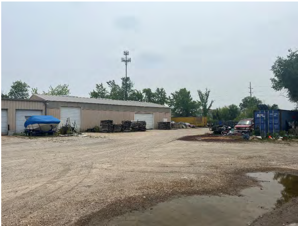
Photo 14 - View of the adjoining property to the east.
