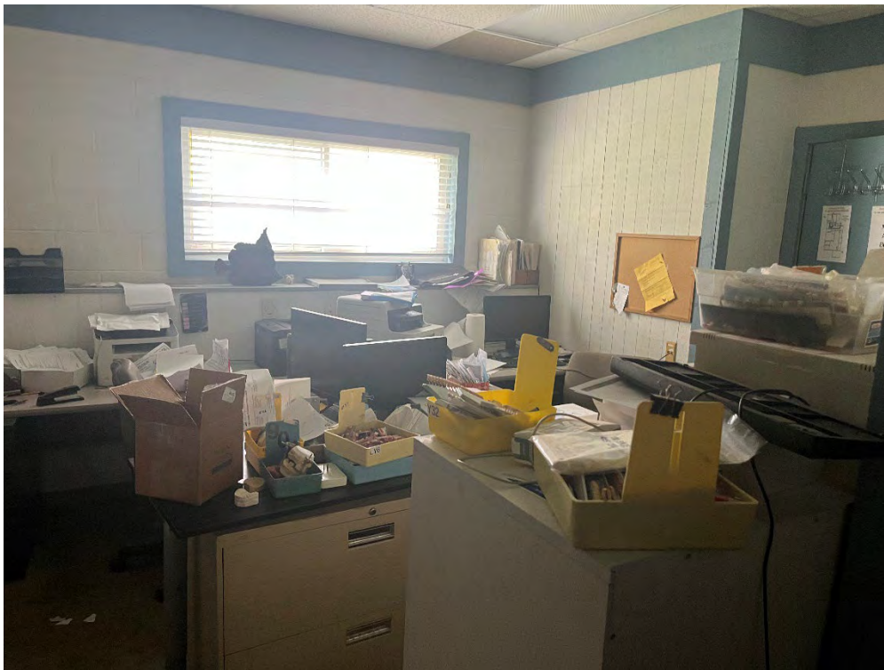
Photo 8 - View of a former office area.
