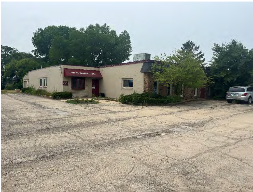
Photo 6 - View of the building, facing southwest.
