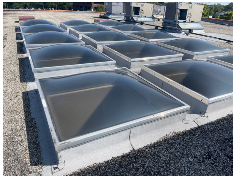
General View of the Skylight(s)
