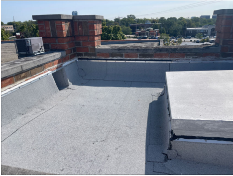
View of Roof
