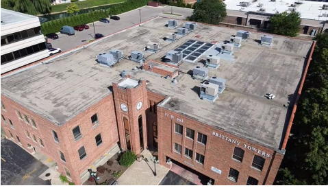
Aerial View of Roof
