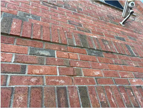
Settlement Cracks
