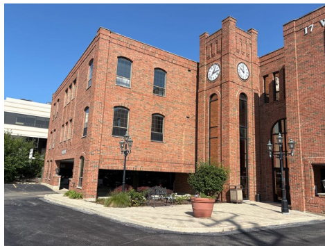
View of Masonry
