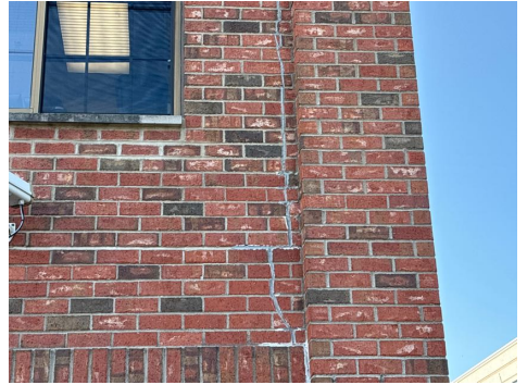
Settlement Cracks
