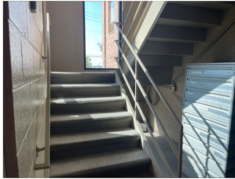
View of Stairs
