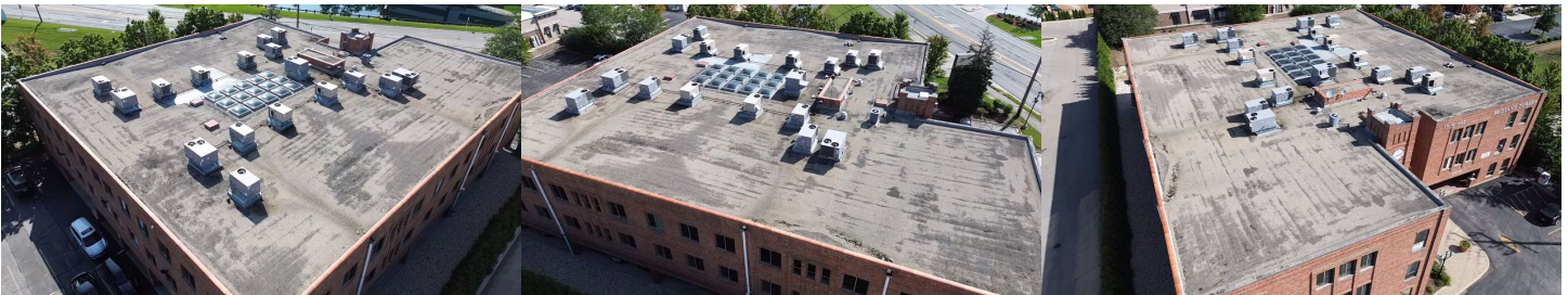
Aerial View of Roof
