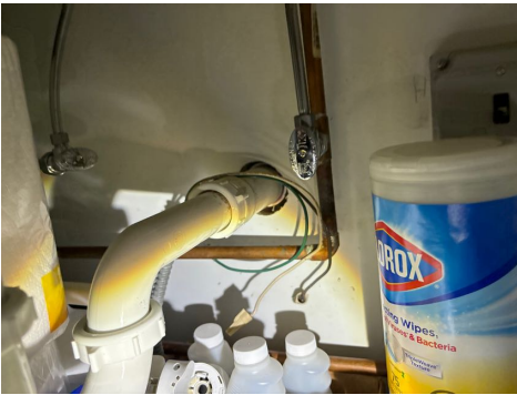
Exposed Splices-Suite 302 Kitchenette
