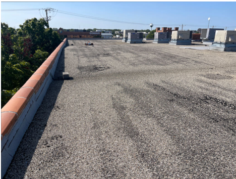
View of Roof
