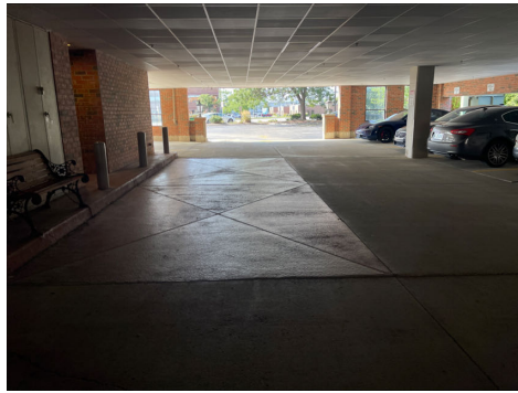
View of Garage Interior
