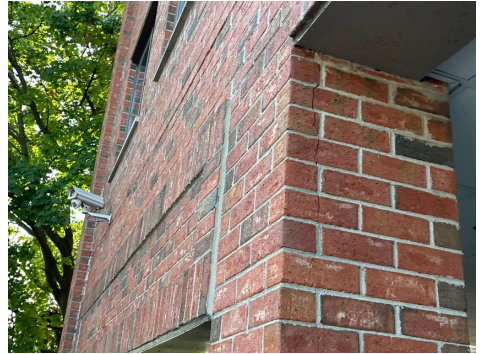
Settlement Cracks
