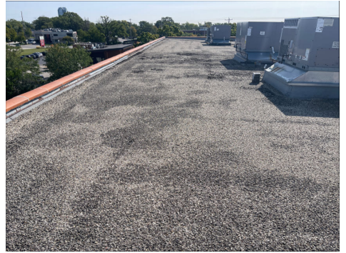
View of Roof
