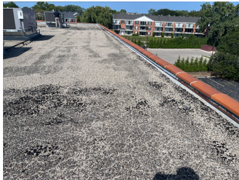
View of Roof
