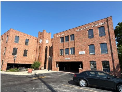
View of Masonry
