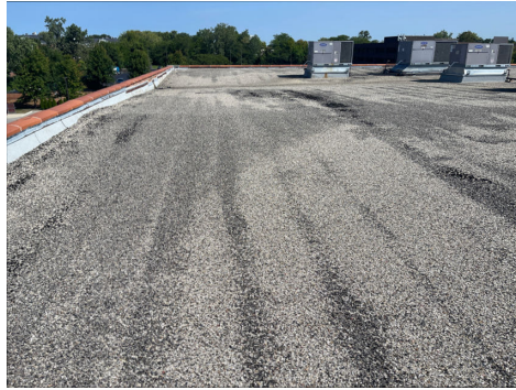
View of Roof
