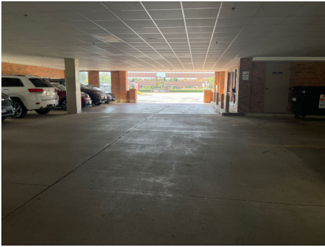
View of Garage Interior
