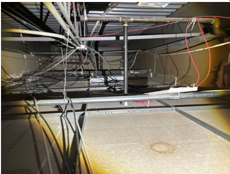
View of Attic Space
