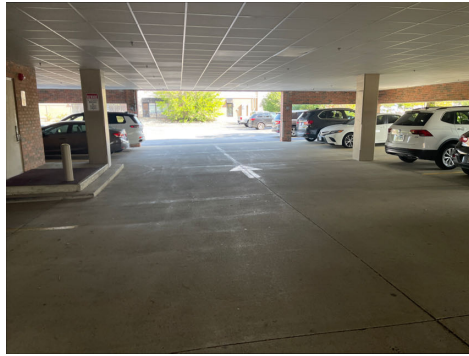
View of Garage Interior
