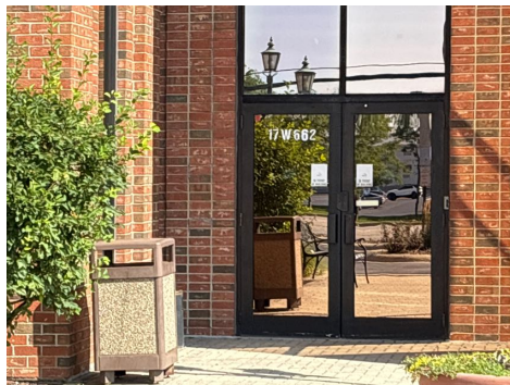
View of Exterior Door
