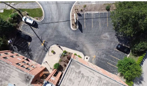
View of parking
