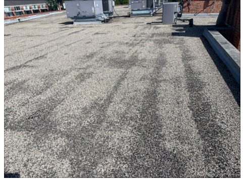
View of Roof
