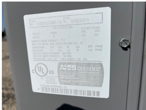
Suite 201 Condenser Data Plate (2016 Allied)
