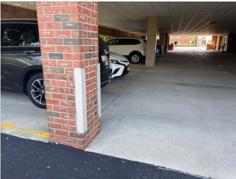
View of corner protection
