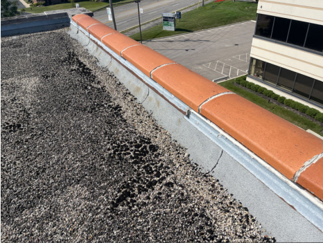
View of Parapet
