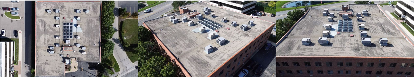
Aerial View of Roof
