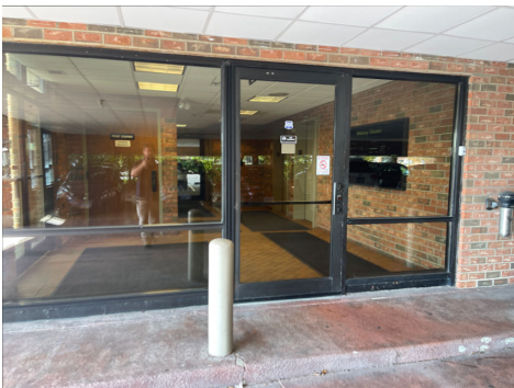
View of Exterior Door
