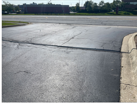
View of access
