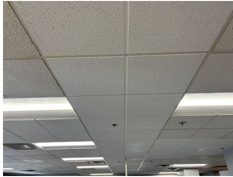
View of Suite 300 Ceiling
