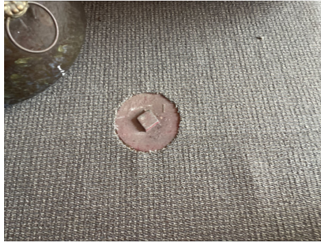
Sewer Clean out-Stairwell
