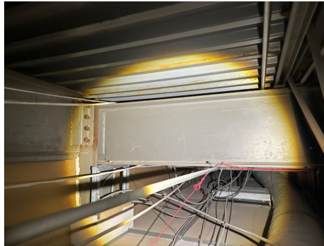
View of Roof Framing
