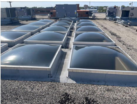
General View of the Skylight(s)
