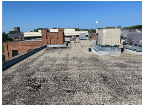
View of Roof
