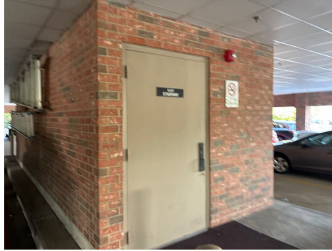
View of Exterior Door
