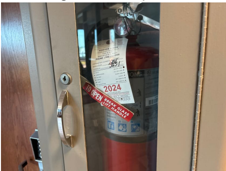
View of extinguisher
