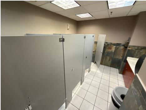
View of 2nd Floor Women's Restroom
