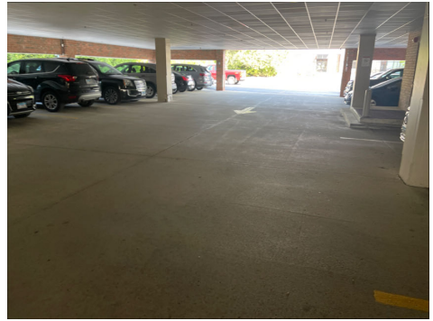
View of Garage Interior
