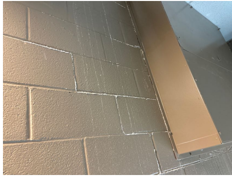
Efflorescence-Stairway
