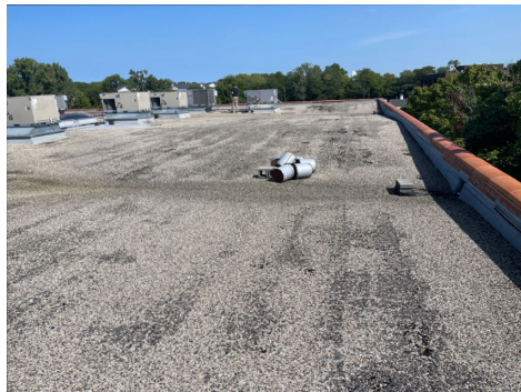
View of Roof
