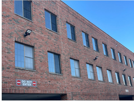
View of lighting
