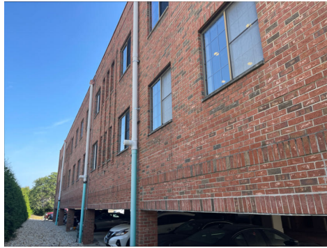
View of Masonry
