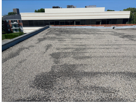
View of Roof
