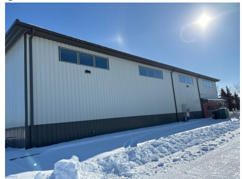
View of Metal Siding
