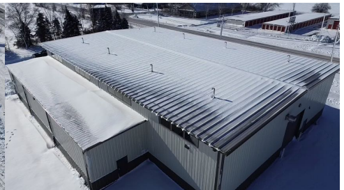
View of Roof
