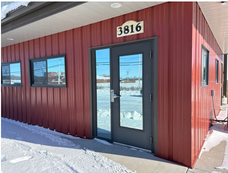
View of Exterior Door
