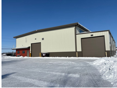
View of Metal Siding
