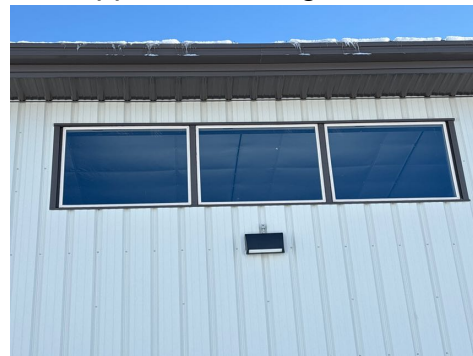
View of windows
