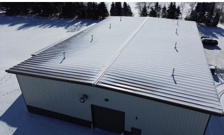
View of Roof
