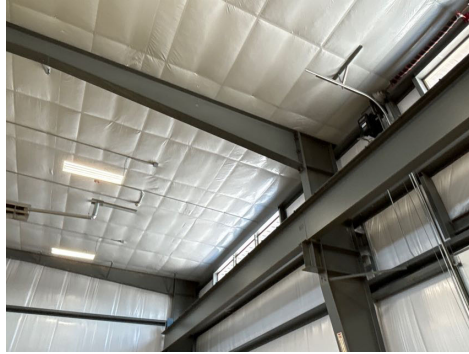
View of Roof Framing
