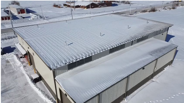
View of Roof
