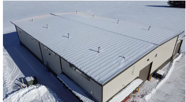
View of Roof
