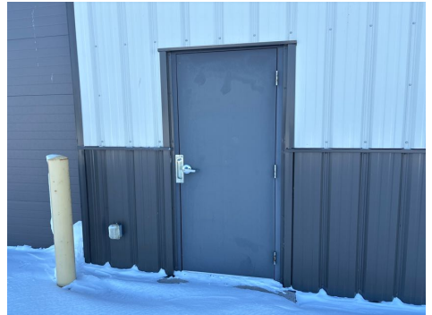
View of Exterior Door
