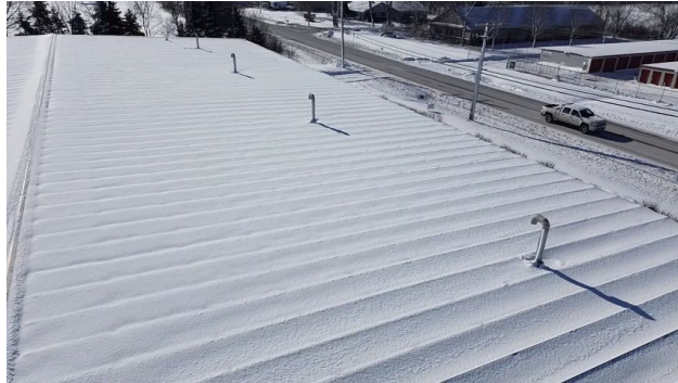
View of Flue Pipes
