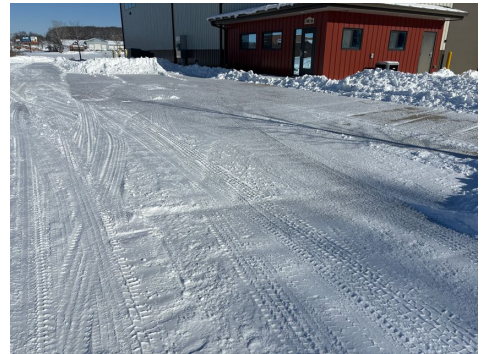
View of parking
