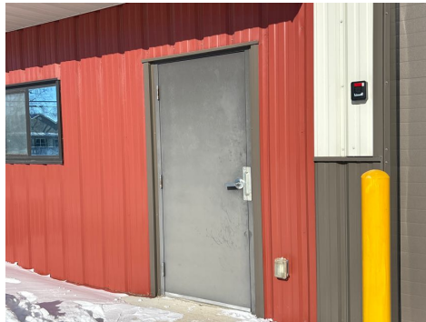
View of Exterior Door
