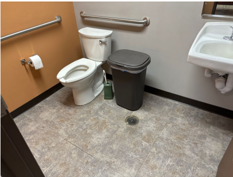
View of Office Restroom
