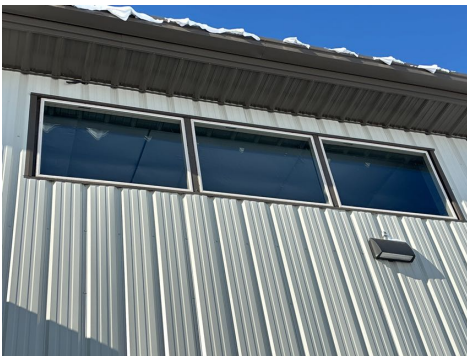
View of windows
