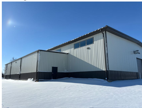
View of Metal Siding
