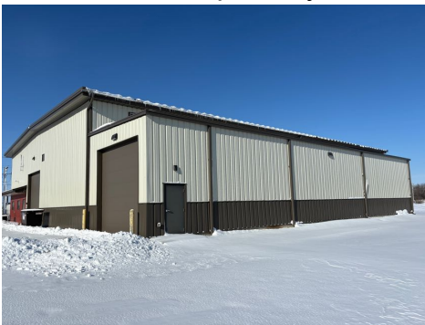
View of Metal Siding
