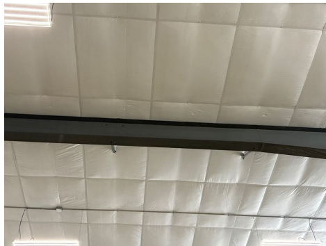
View of Sheathing
