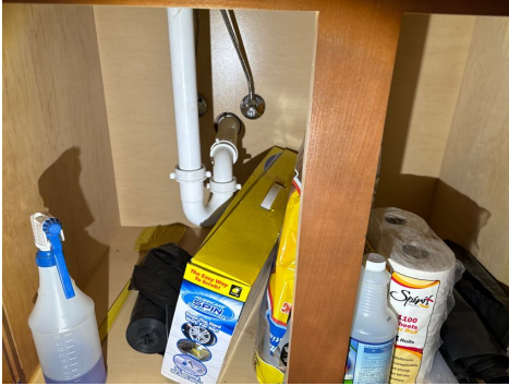
General View of Sink Drain
