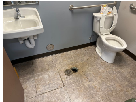
View of Warehouse Restroom
