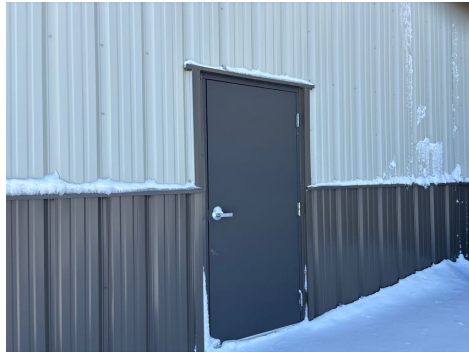
View of Exterior Door
