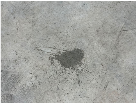
2nd Infrared Heater Drip
