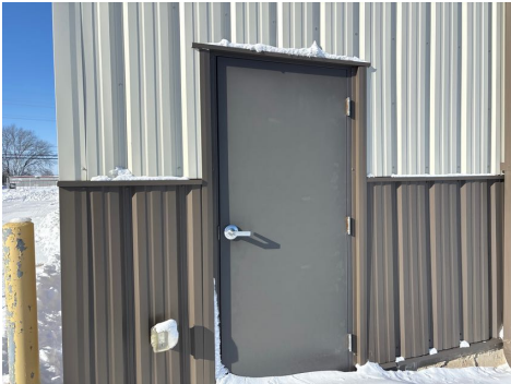
View of Exterior Door
